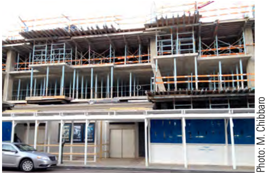
Figure 13.12. A typical 4 ft.-wide temporary walkway (painted white) over a sidewalk adjacent to a construction site. The wide span between posts accommodates the double exit doors (shown in the center), which serve an occupied cinema.
