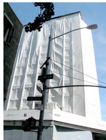
Figure 13.16. A temporary barrier covering an entire building.
