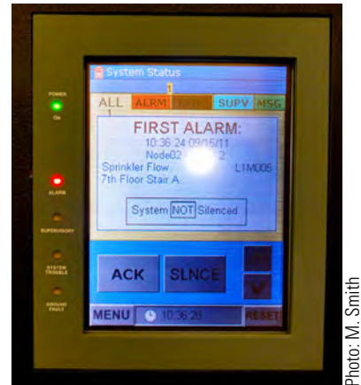
Figure 11.3 A textual-style annunciator panel with a touch-screen display.
