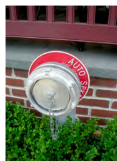
Figure 10.5. A quick-connect type of FDC.
