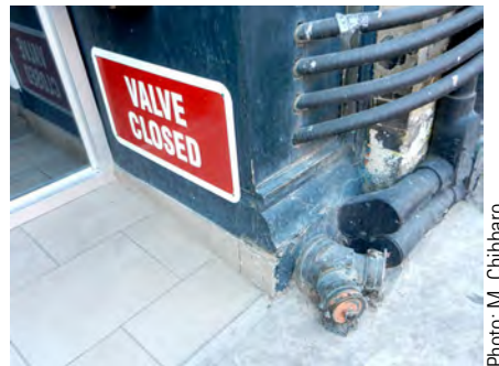
Figure 13.15. A sign next to an FDC indicating that the system valve is shut off.
