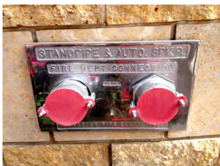
Figure 10.3. A combined sprinkler and standpipe FDC.
