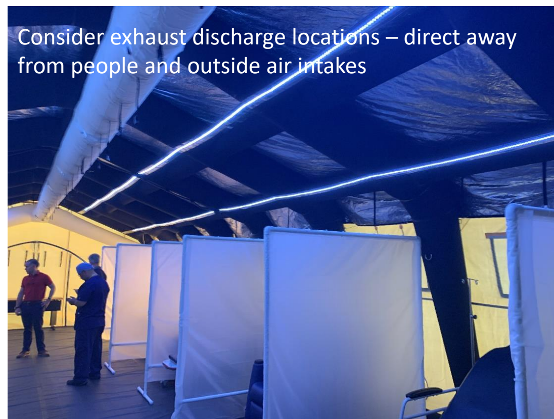
Bottom opening exhausted to create front to back airflow across patient
