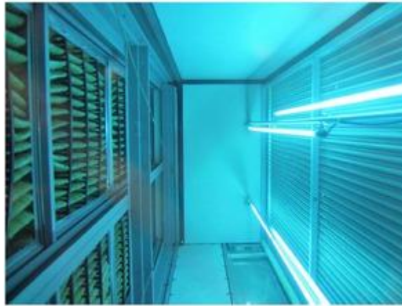
Figure 9. In-AHU Air and Surface Disinfection (Bahnfleth 2020)
