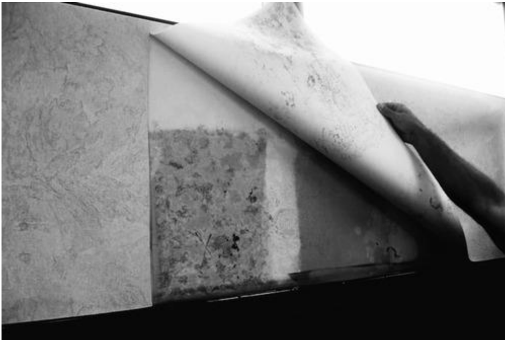
Figure 5. Impermeable Vinyl Wall Covering on Exterior Wall
