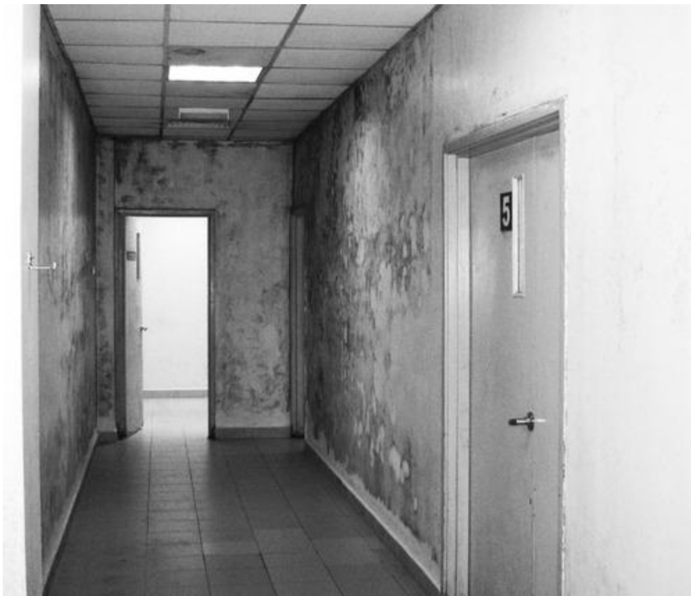
Figure 7. Mold Resulting from Humid Air Infiltration in Overcooled Health Clinic
