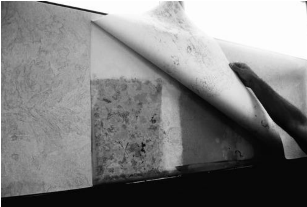
Figure 5. Impermeable Vinyl Wall Covering on Exterior Wall
