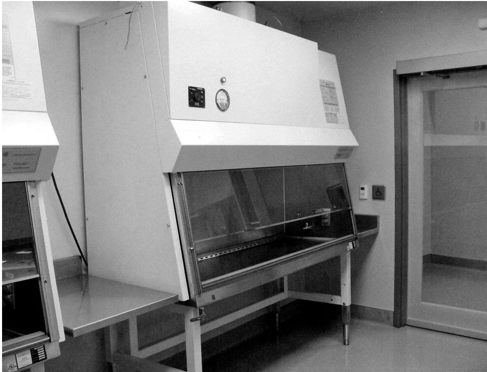
Figure 8-15 ISO 5 Biological Safety Cabinet in ISO 7 Chemotherapy Mixing Room
