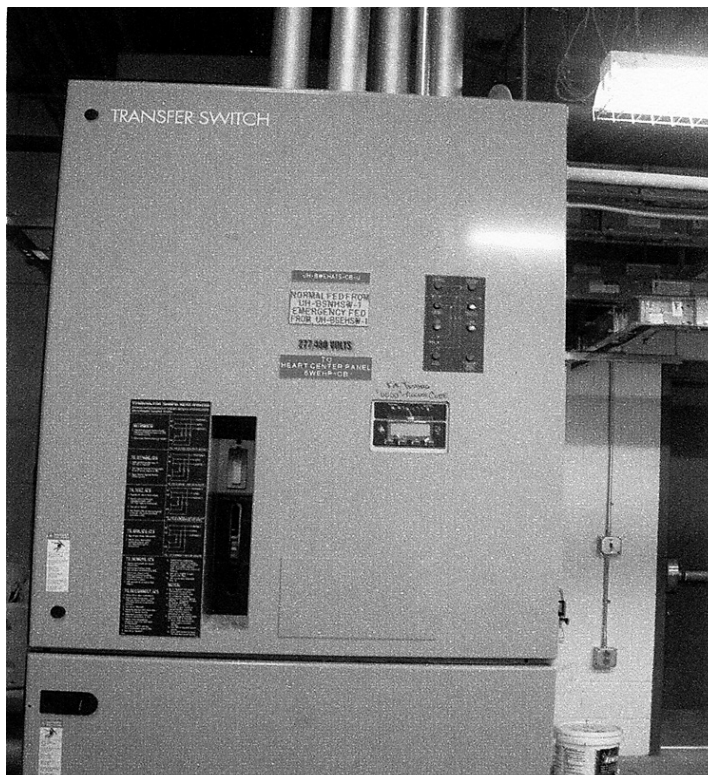
Figure 10-3 Emergency Load Transfer Switch
