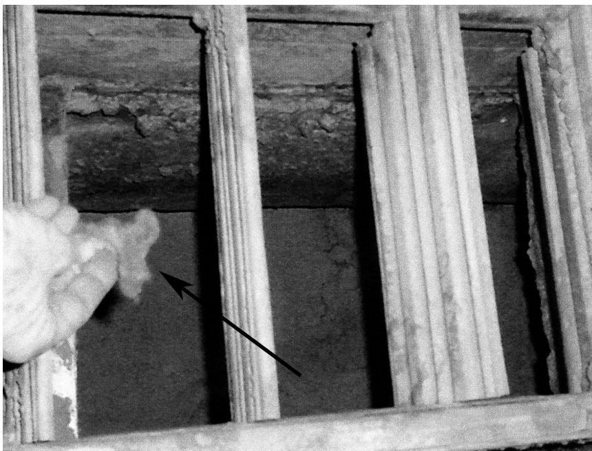
Figure 7-6 Ductwork Lining Peeling off into Airstream
