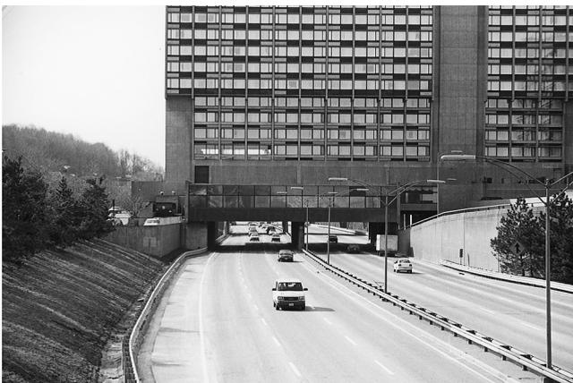
FIGURE A.3.3.49.1 Air-Right Structure.
