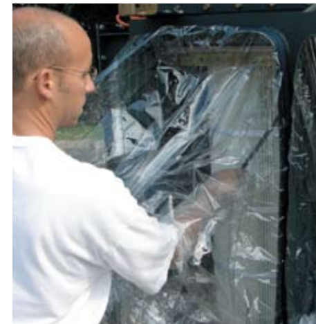
Hazardous compounds contained with BIBO filter change. Filters are sealed via cam-lock action, making it easy to work through the bag.
