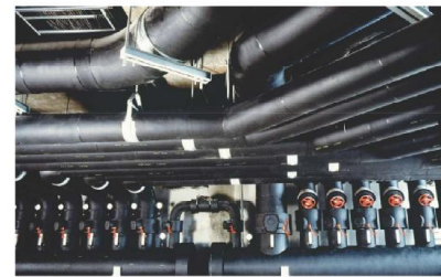
Many advantages described above making Aeroflex suitable for insulating chilled water piping.
