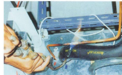
Self-extinguished property, low smoke density, less toxic gases and non-melting characteristic when burnt, making Aeroflex widely used in air-conditioning systems.
