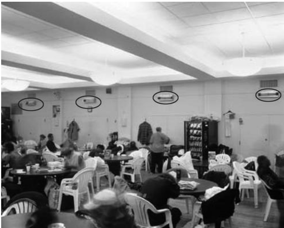
Figure 9. Upper-Room UVC (Circled) Treating Congregate Setting (TUSS Project, St. Vincent's Hospital, New York City)
