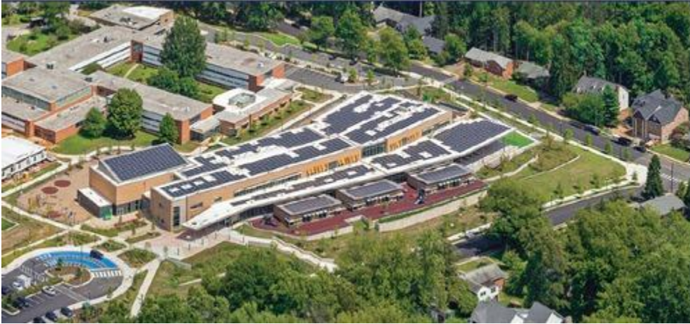
Figure 22. PV Installation at Discovery Elementary, Net Zero Energy School, Arlington, VA: 500 kW (Beaufait 2018)
