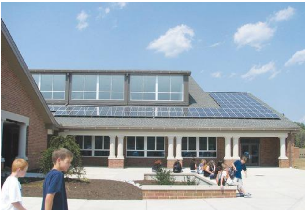
Figure 21. Example of PV Installation at Twenhofel Middle School, Independence, KY: 22 kW (Seibert 2010)
