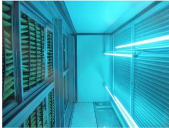
Figure 9. In-AHU Air and Surface Disinfection (Bahnfleth 2020)
