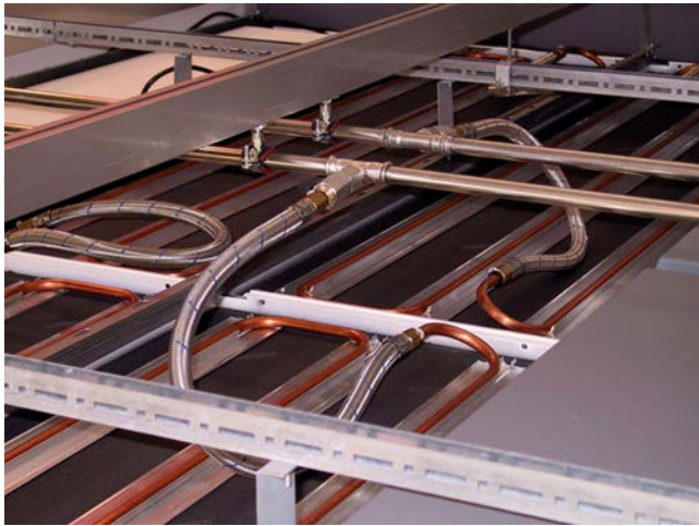
Fig. 3 Back View of Drop Ceiling: Piping Configuration with Flexible Hose and Quick-Connect Fittings
