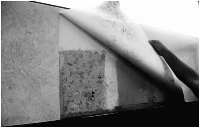
Fig. 4 Impermeable Vinyl Wall Covering on Exterior Wall
